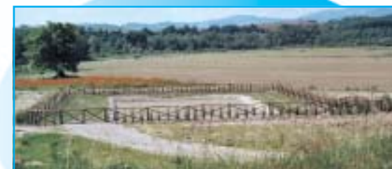
Already existing constructed wetland similar to the one designed for Sellustra Life (photo Iridra srl)
