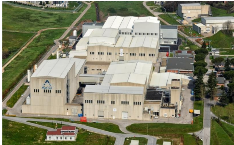
Booster Case Facilities
